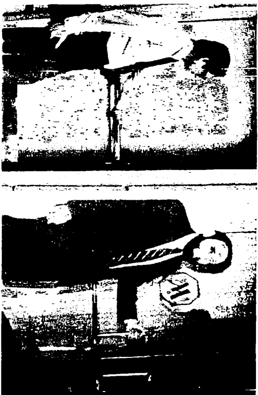
1.5 Affordances of Doors. Door hardware can signal whether to push or pull without signs. The flat horizontal bar of A (above left) affords no operations except pushing; it is excellent hardware for a door that must be pushed to be opened. The door in B (above right) has a different kind of bar on each side, one relatively small and vertical to signify a pull, the other relatively large and horizontal to signify a push. Both bars support the affordance of grasping: size and position specify whether the grasp is used to push or pull—though ambiguously.
